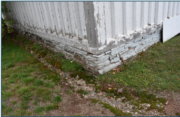
Figure 6: Drainage ditch on north side
