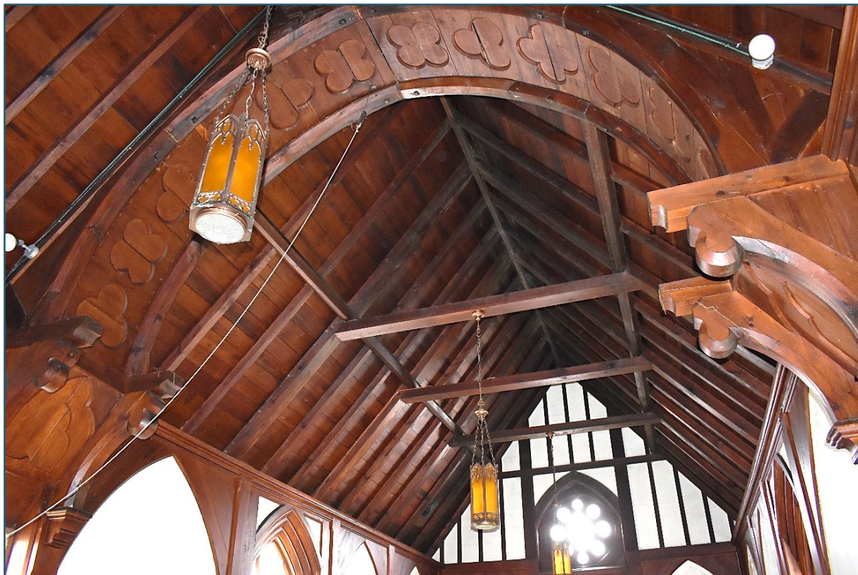
Figure 23: St. Mary the Virgin Catholic Church interior roof structure
