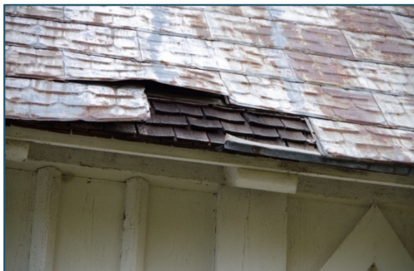
Figure 19: Original wood shingles under newer metal roof
