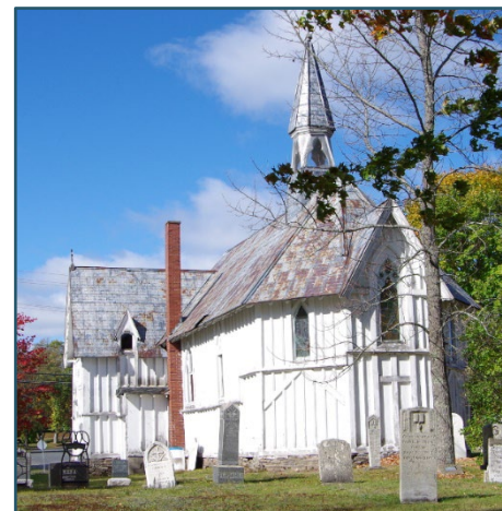
Figure 3: East gable, showing stained glass, cross motif, and trefoiled bell tower
