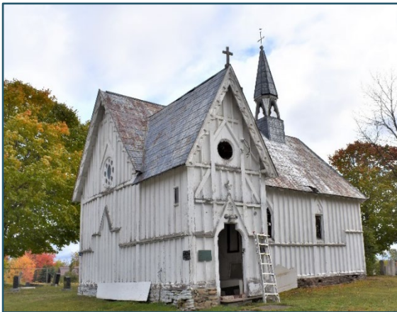
Figure 32: Decorative wood detailing on west and south facades
