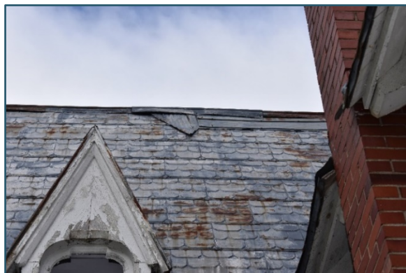
Figure 21: Patched roof at previous chimney location
