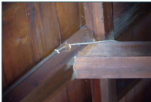
Figure 22: Pegged mortice and tenon joint between rafter and tie beam
