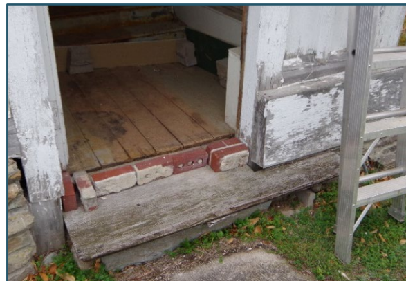
Figure 10: Stone door sill, removed
