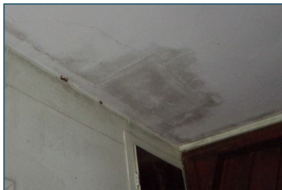
Figure 46: Previous chimney hole in narthex ceiling
