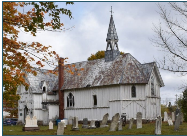
Figure 33: Southeast view, showing wood detailing around apse
